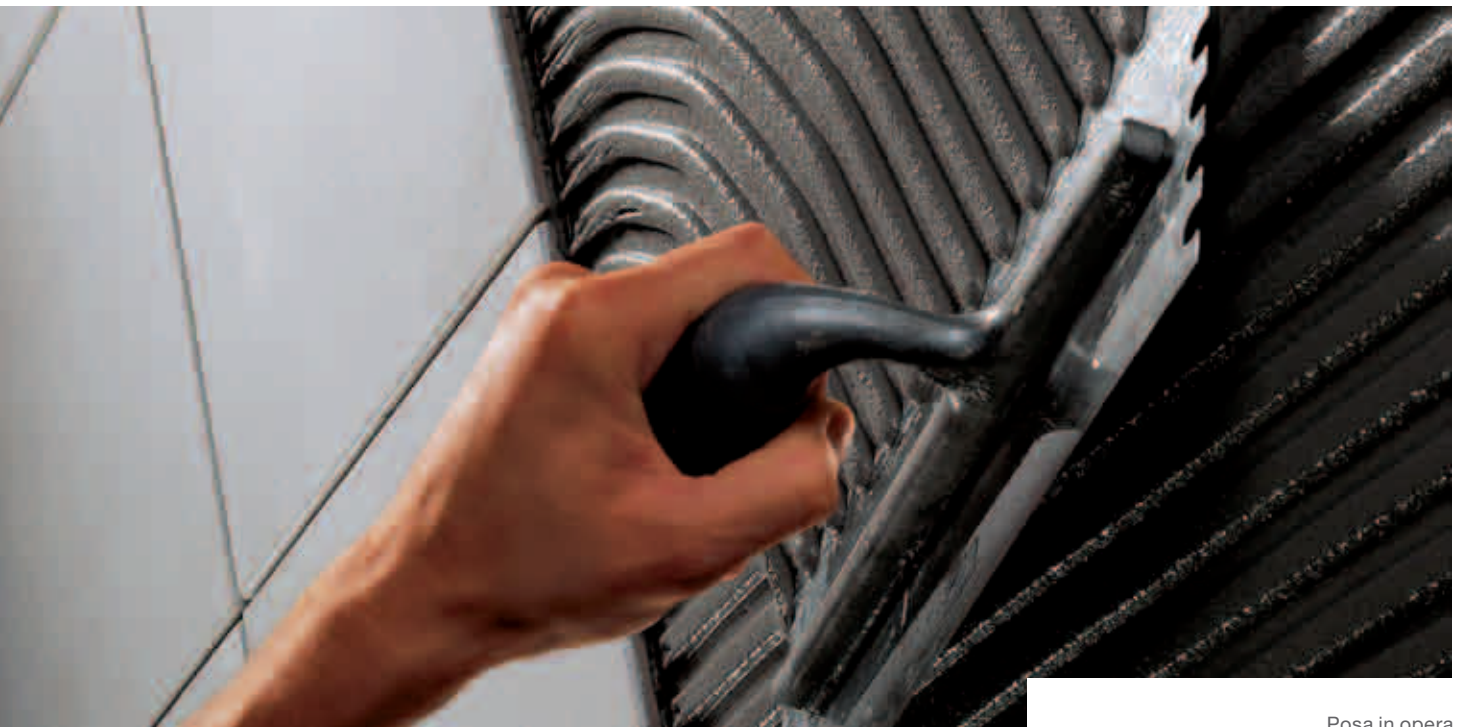
Posa in opera
