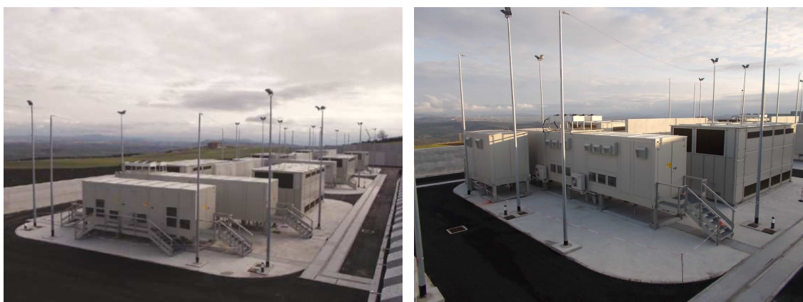
Fig.3: Impianto Large Scale Energy Intensive 12MW/80MWh – Ginestra SANC presso Castelfranco in Miscano (BN)
