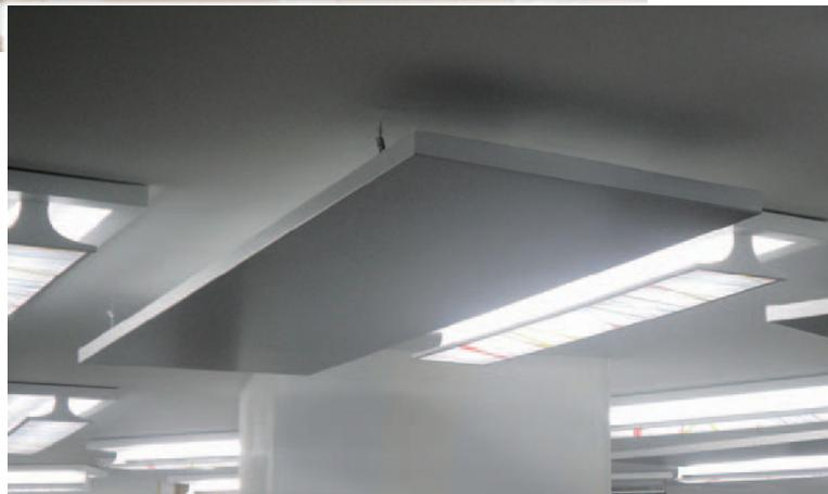
**T**he panel can be supplied with hot or cold water: in the summer, it should be used together with a primary air system, as only sensible cooling is provided.
