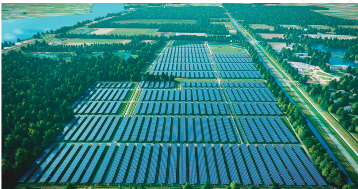
35 MW solar Carport, Dronten, Netherlands.
