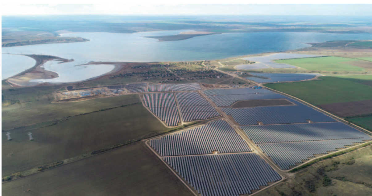
148 MW, Progressovka plant, Mykolayiv, Ukraine.
