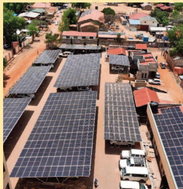
The new carport off-grid system for UAP Old Mutual Equatoria Towers, Juba, Sudan.
